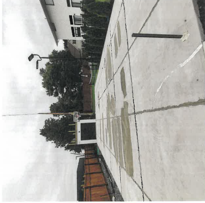
1. Clean Court Surface, Repair Cracks if Applicable
