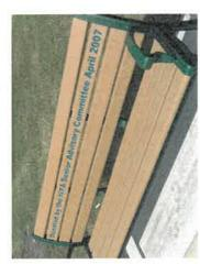
The bench slats are constructed from recycled plastic materials and backed by a 50 year warranty. The legs are made of coated aluminum. Regular maintenance will be completed on the legs, due to weathering.
