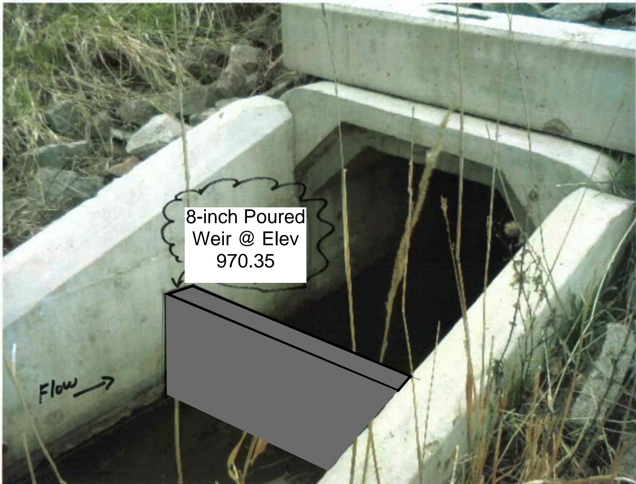
Figure 4. Concept design of Barnes Lake outlet weir.
