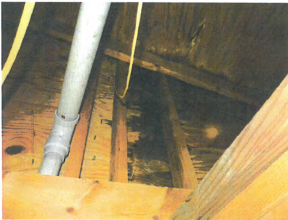
Photograph #6 – Staining below roof/wall intersection
