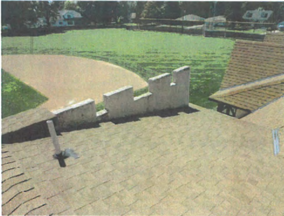
Photograph #7 – Stucco parapet walls
