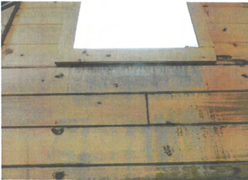
Photograph #4 – Staining below window at north wall
