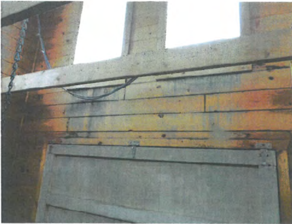
Photograph #5 – Staining below windows at south wall
